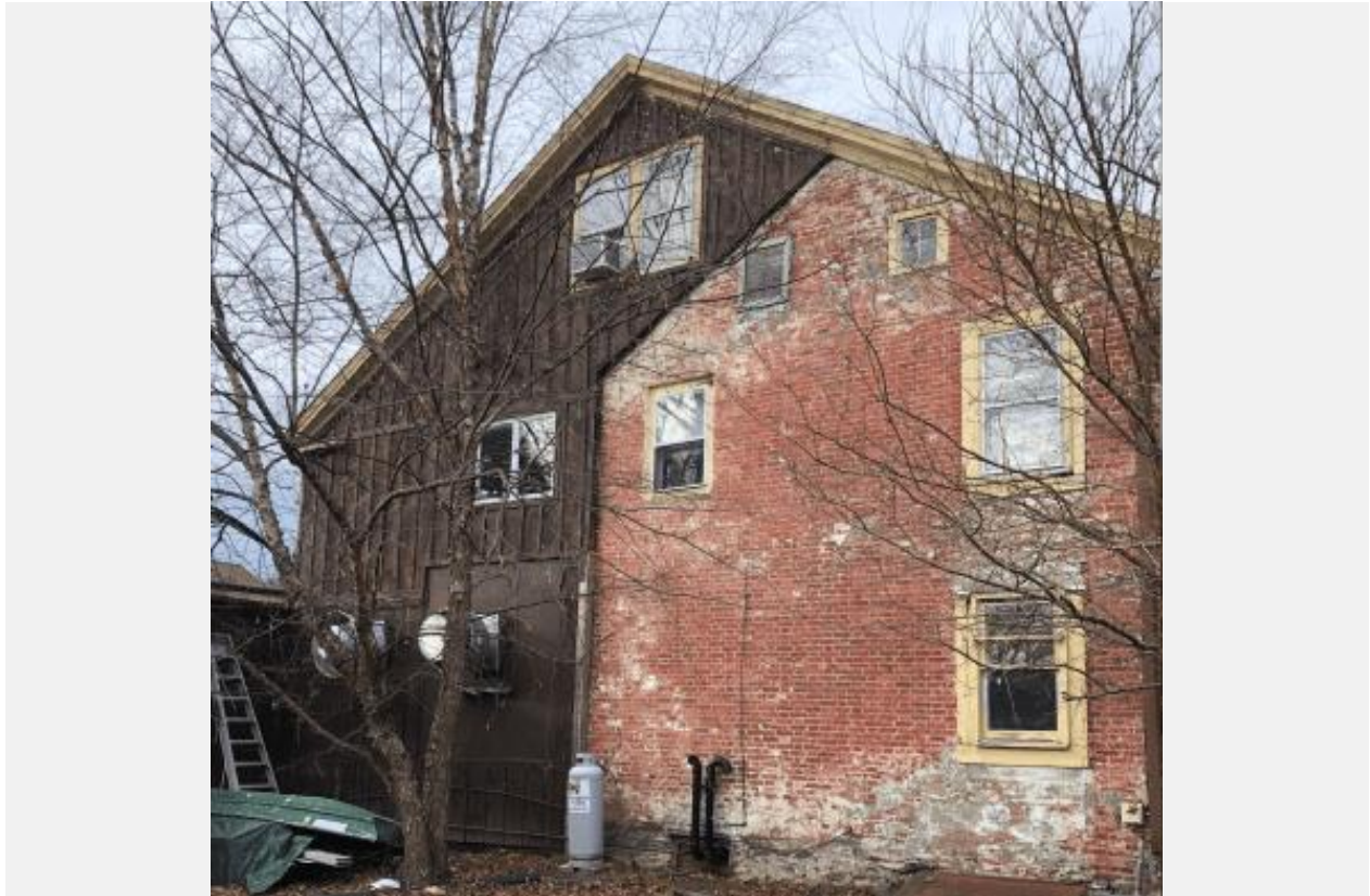
East end of the Hillsdale House. The vestiges of the original (brick) R. Latting Tavern are still visible.
