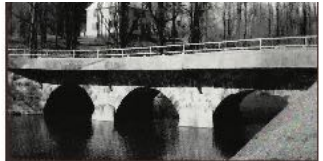
The three-span stone Ancram Paper Company Bridge over the Roeliff Jansen Kill was built in 1850. It is recognized as the oldest known bridge in Columbia County. (1937) A 1937 postcard of the Old Stone Bridge at Ancram. (1989) A more contemporary photo of the bridge from the book "Looking for Work in Columbia County" by Peter Stott (1989/90)
